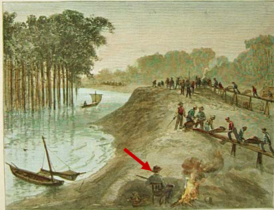
BUILDING A LEVEE.
